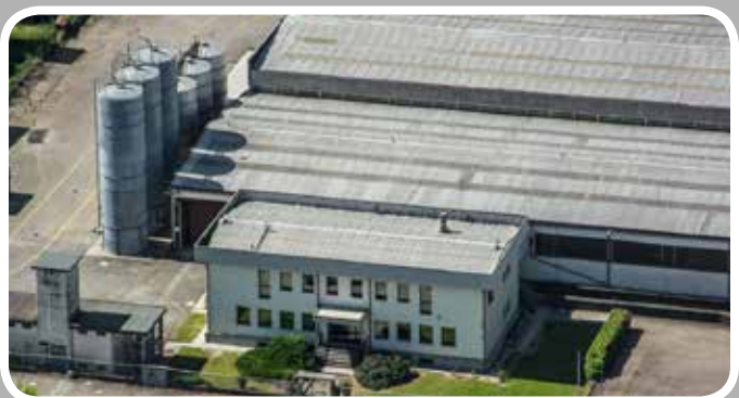
Production Centre - Imola (BO) - Italy
